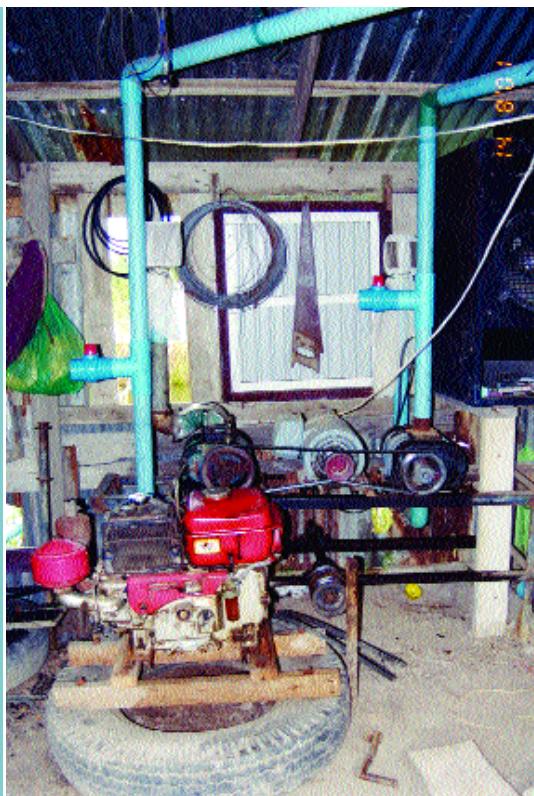
Figure 28 Power supplies are not always reliable. Loss of aeration can quickly cause devastation in a hatchery. This hatchery has not only installed two electrically-driven blowers (one as a back-up) but has also provided a petrol engine so that the drive belts can be rapidly changed if the power fails (Thailand)
