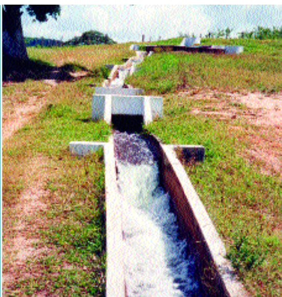
Figure 53 Where the topography of the site makes it feasible, supplying water by gravity keeps the dissolved oxygen level high (Brazil)
